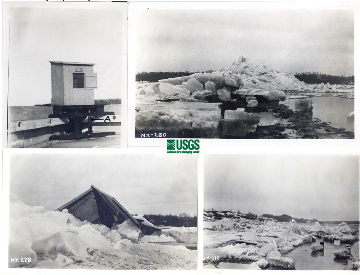
Fig 1. United States Geological Survey gauge house, Lock 7, Mohawk River, before and after the 1914 ice jam.
