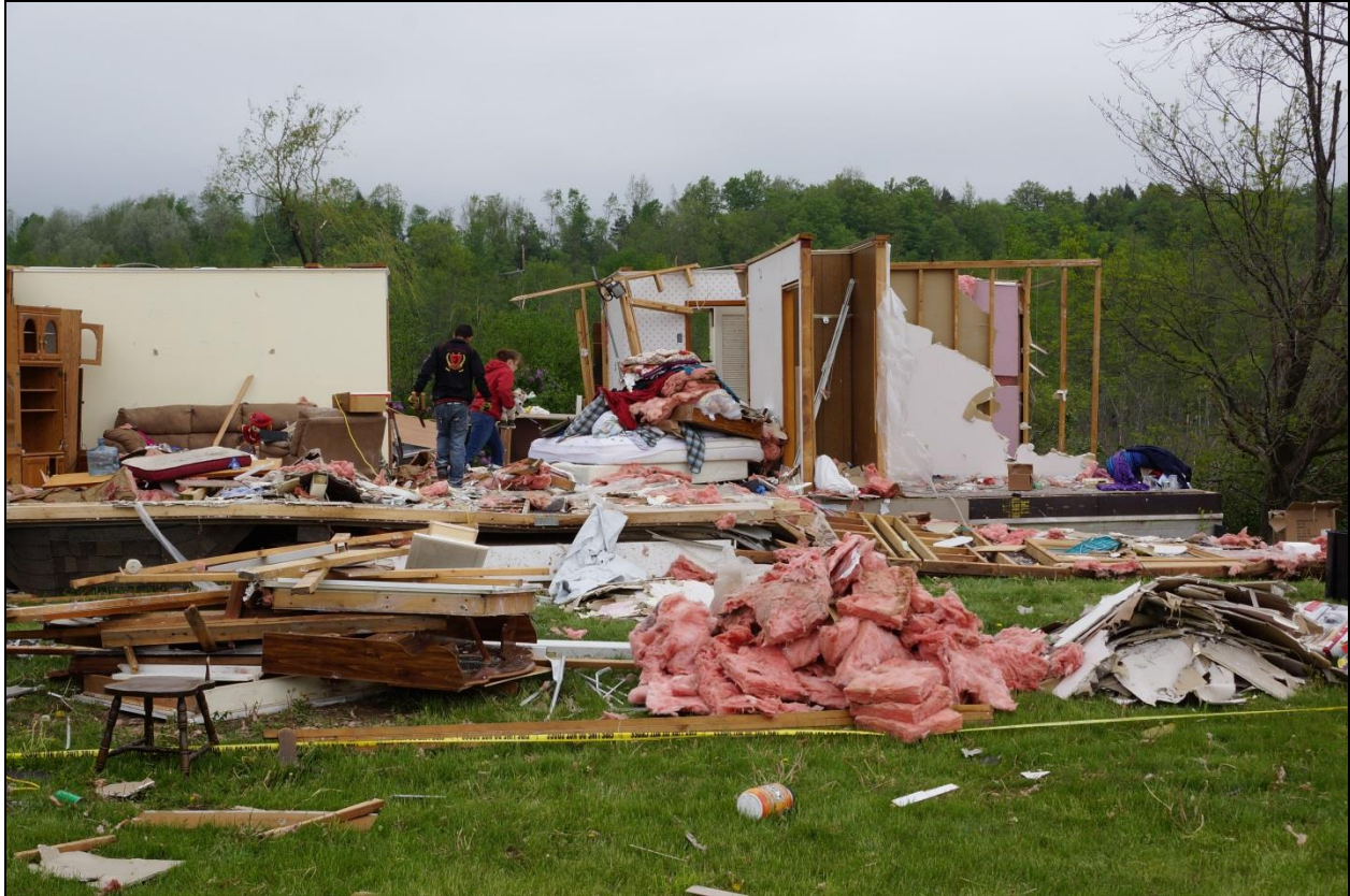
Figure 3: A home situated along State Route 20 in the Town of Duanesburg, almost completely destroyed. Only one wall remained standing after the tornado ( NWS at Albany image ).
