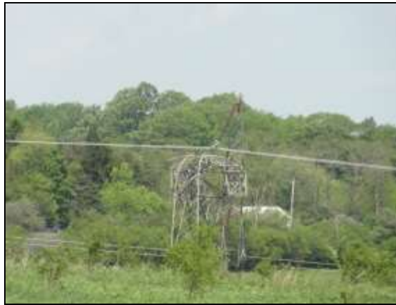
Figure 4: Extensive tornado tree damage viewed along a ridge line in Schoharie County from the junction of Dutch Hill and Wharton Hollow Rds. Photo Source: NWS Albany
