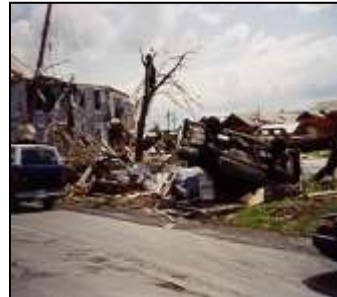
Figure 5: F3 damage from the Mechanicville Tornado of May 31, 1998 (NWS at Albany photograph).
