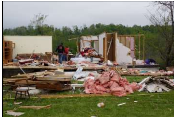
Figure 3: A home situated along State Route 20 in the Town of Duanesburg, almost completely destroyed. Only one wall remained standing after the tornado ( NWS at Albany image ).
