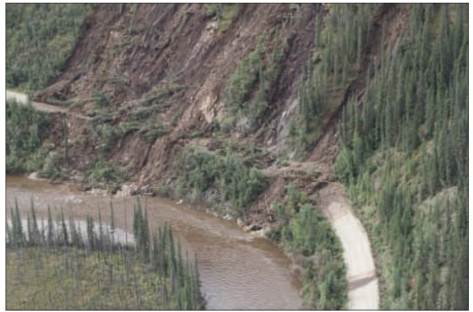
Taylor Highway near Milepost 115 and O'Brien Creek This landslide was approximately 750 feet long and covered with debris 20 feet thick
