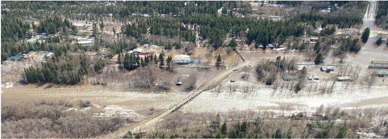
Fig 3: Many buildings in the community had water in or around them. The bridge over Manley Slough was within six inches of being overtopped.
