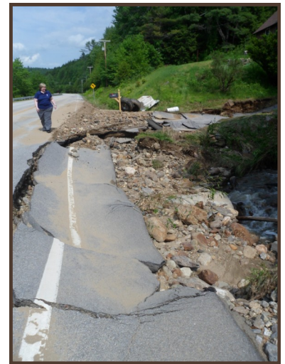
Above: Road damage on Route 9 in NH due to flash flooding on May 29 th .
