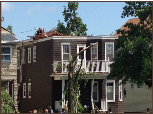
Above: Tornado Damage in Revere, MA on July 28th. Photo taken by Marek Kozubal
