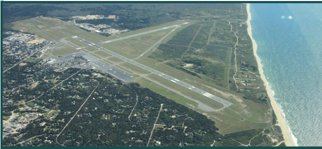
Nantucket Airport —Located on the south central portion of the Island.
