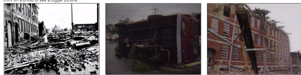
Above: A four-story, jewelry manufacturing building in Providence that had its top story blown off by the tornado. Photo in NOAA Archives courtesy of the Providence Journal. Above: A truck flipped by the 1986 Cranston-Providence tornado. Picture courtesy of T.J. Del Santo and WPRI-TV. Above: Fulford Manufacturing Building after the 1986 tornado hit it. Picture courtesy of T.J. Del Santo and WPRI-TV.
