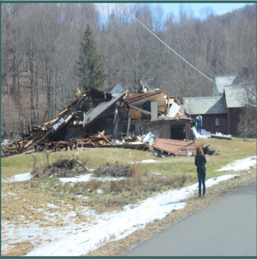
Above: Conway Massachusetts tornado damage Photo by: W1NWS-Ray Weber and Alex Kamyshin
