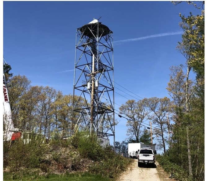
Radome being lifted off of the pedestal
