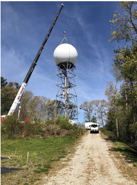
Radome being lifted off of the pedestal
