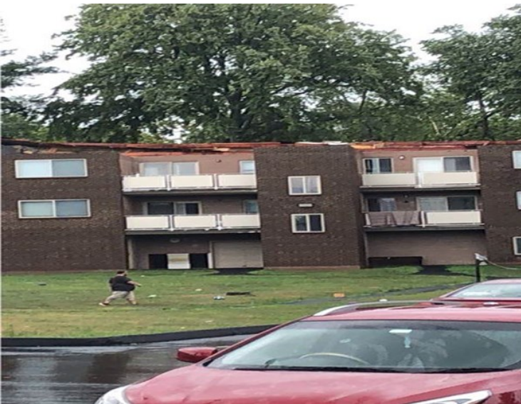
Roof torn off an apartment complex in Wethersfield, CT. Photo by Jim Peruta (KC1JDP).
