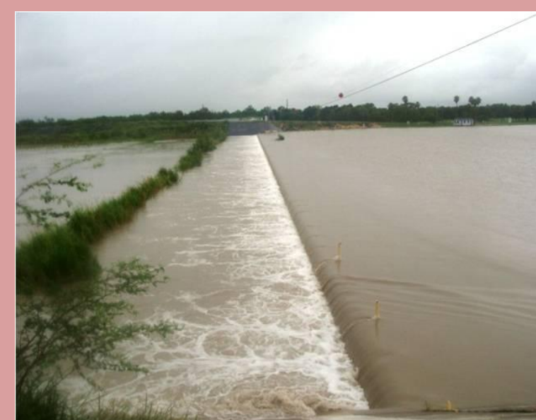
Banker floodway after diversion at Anzalduas on 8 July 2010
