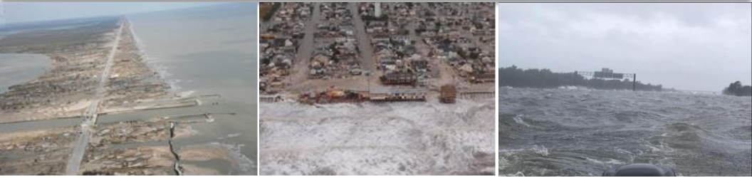
Left: Bolivar Peninsula scraped clean by Ike's Storm Surge in 2008. Center: Damaged and destroyed homes along the Jersey Shore from Sandy in 2012. Right: Interstate 10 along Jefferson/Chambers Co. Line in 2017 during Harvey.
