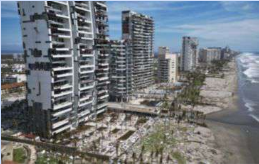
Above: Hollowed-out high rise hotels and condos at Acapulco Beach. Photo courtesy of AFP/Getty Images
