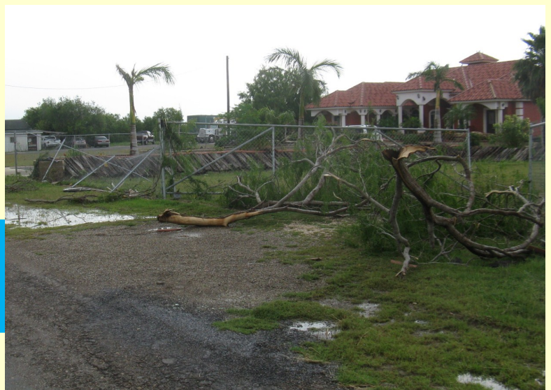
Right: A tornado containing 80 mph winds damaged property and portions of a large single family home early on May 11th, 2012 in San Benito , TX.
