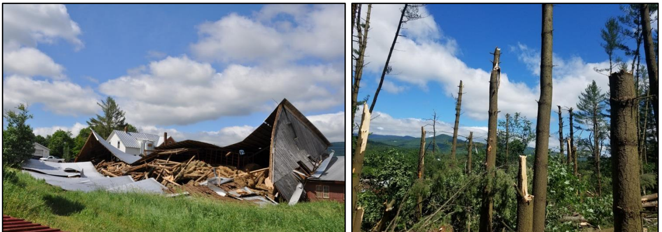
Figure 7: Collapsed hay barn (left) and snapped pine trees (right) 1 mile south-southeast of Waitsfield, VT. Pictures from NWS Storm Damage Survey.
