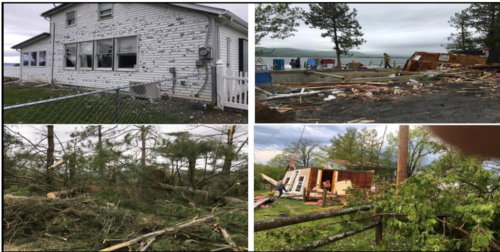
Figure 6: Storm survey photos taken by NWS BTV on Potash Bay Road in Western Addison County.
