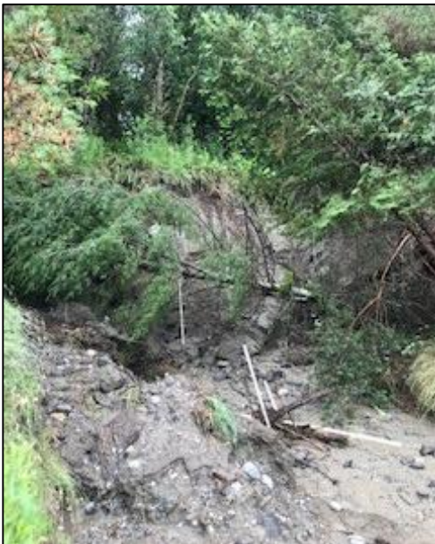
Figure 5 (left). Mud Slide that occurred in St. Johnsbury. Pictures courtesy of State of Vermont, Division of Fire Safety.
