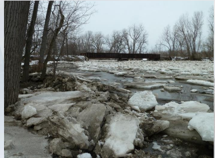
Buffalo Creek railroad crossing between Union and I-90 on March 17, 2015
