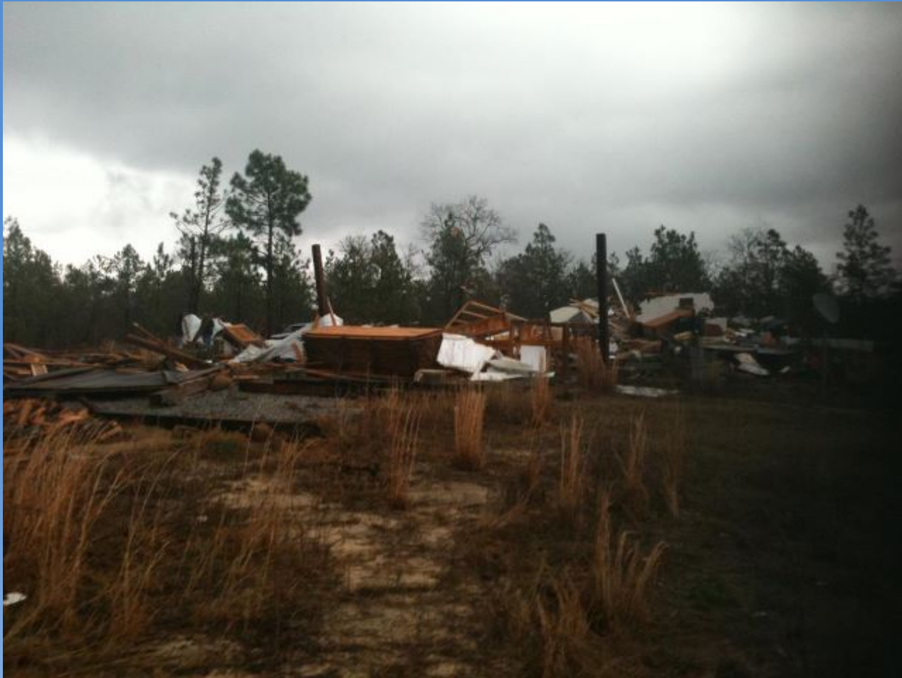
Damage associated with the tornado near Wagener
