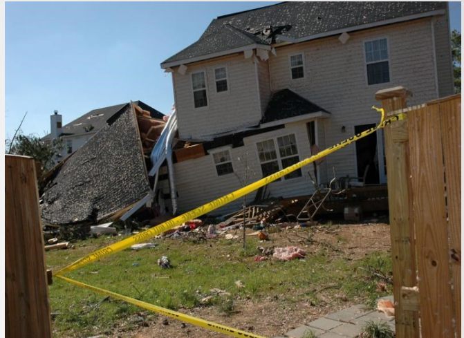
EF3 damage to homes in Newberry County
