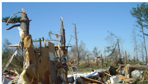
A mobile home destroyed by an EF2 Tornado near Prosperity, SC
