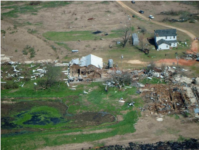
EF2 damage to dairy farm in Burke County
