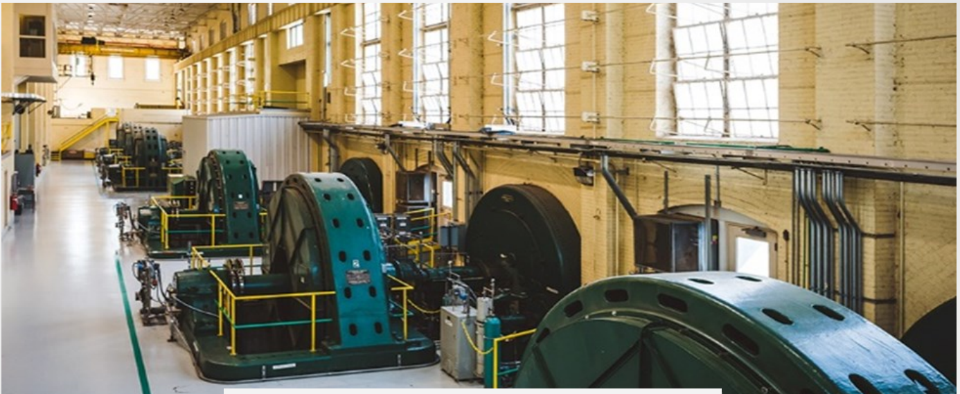
View from inside the Blewett Falls powerhouse
