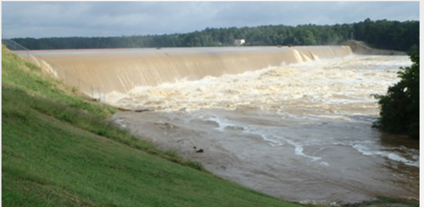
Water flowing over the Blewett Falls Dam during the flooding produced by Hurricane Florence
