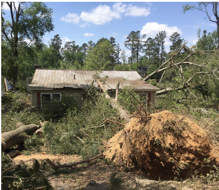
EF-2 tornado damage in Burke County, GA from the April 13, 2020 storms
