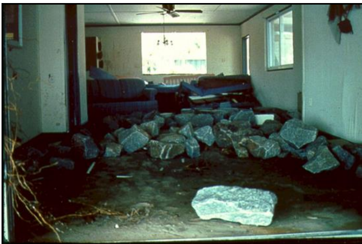
Large rocks deposited into a beachfront home on Folly Beach, SC from Hurricane Hugo's storm surge. [Image courtesy of NWS]
