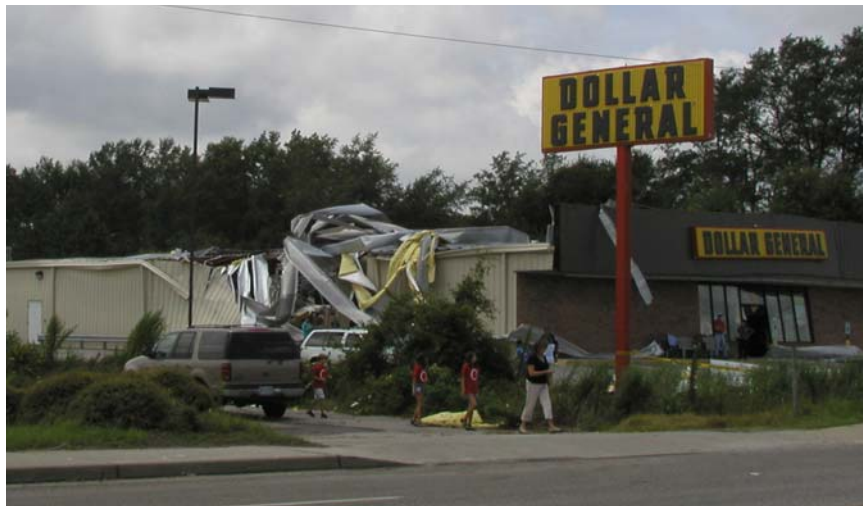
Fig 10. F1 tornado damage in the town of Hampton South Carolina
