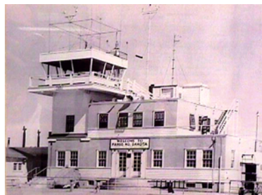
d) Airport Administration Building, Fargo, ND
