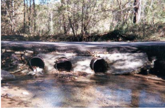
ter Crossing Prior To Mitigation
