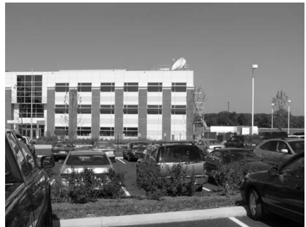
Above is a picture of new office building at Innovation Park. We will be occupying a portion of the third floor. Note the satellite dish on the roof is the main satellite dish through which we obtain all our weather data.
