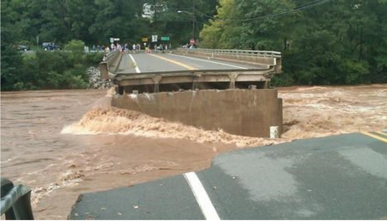
The washed out PA 973 bridge over Loyalsock Creek near Loyalsockville. Image courtesy PA State Police.
