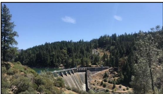
Scott Dam on the Eel River with Lake Pillsbury on the left
