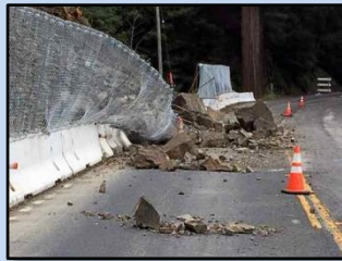
Rockslide fully closed Highway 101 north of Leggett, 3/10/17 [courtesy Caltrans District 1]
