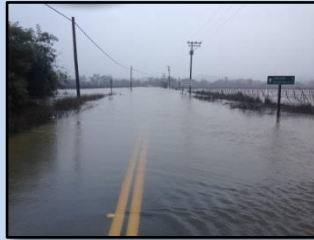
Highway 175 bridge across the Russian River in Hopland closed due to flooding, 1/10/17
