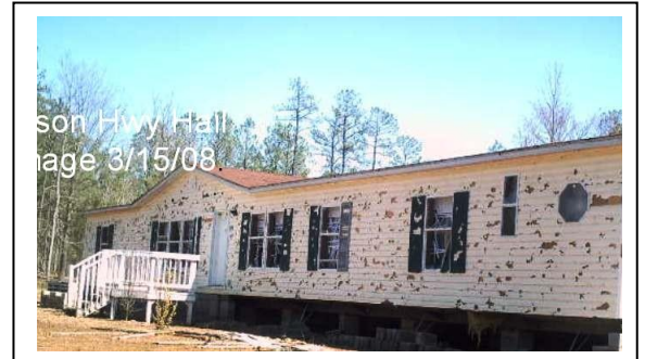
Fig. 9. Another major hazard associated with downbursts is from wind-driven large hail, which can cause injury and major property damage, such as with this manufactured home. Photo courtesy of Greenwood County Emergency Management.
