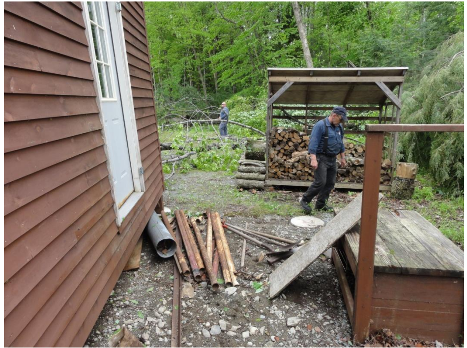
Figure 2: This fishing camp on Sandy Pond was moved six feet off its foundation due to the tornado. The steps on the right in this image used to lead to the door on the left. Photo by NWS Gray, ME.
