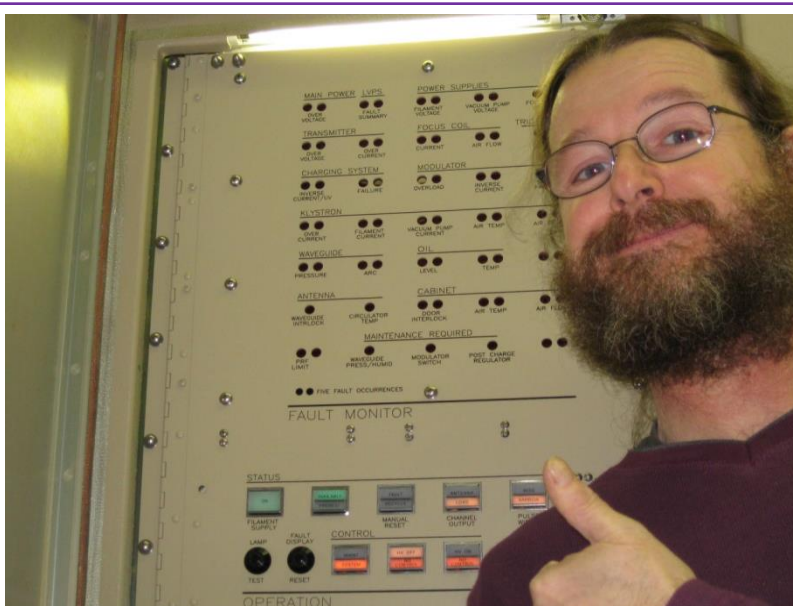
Figure 5: Scott Chick works as an Electronic Technician and helps maintain the office equipment. He is also heavily involved in maintenance on the WSRD 88D radar.
