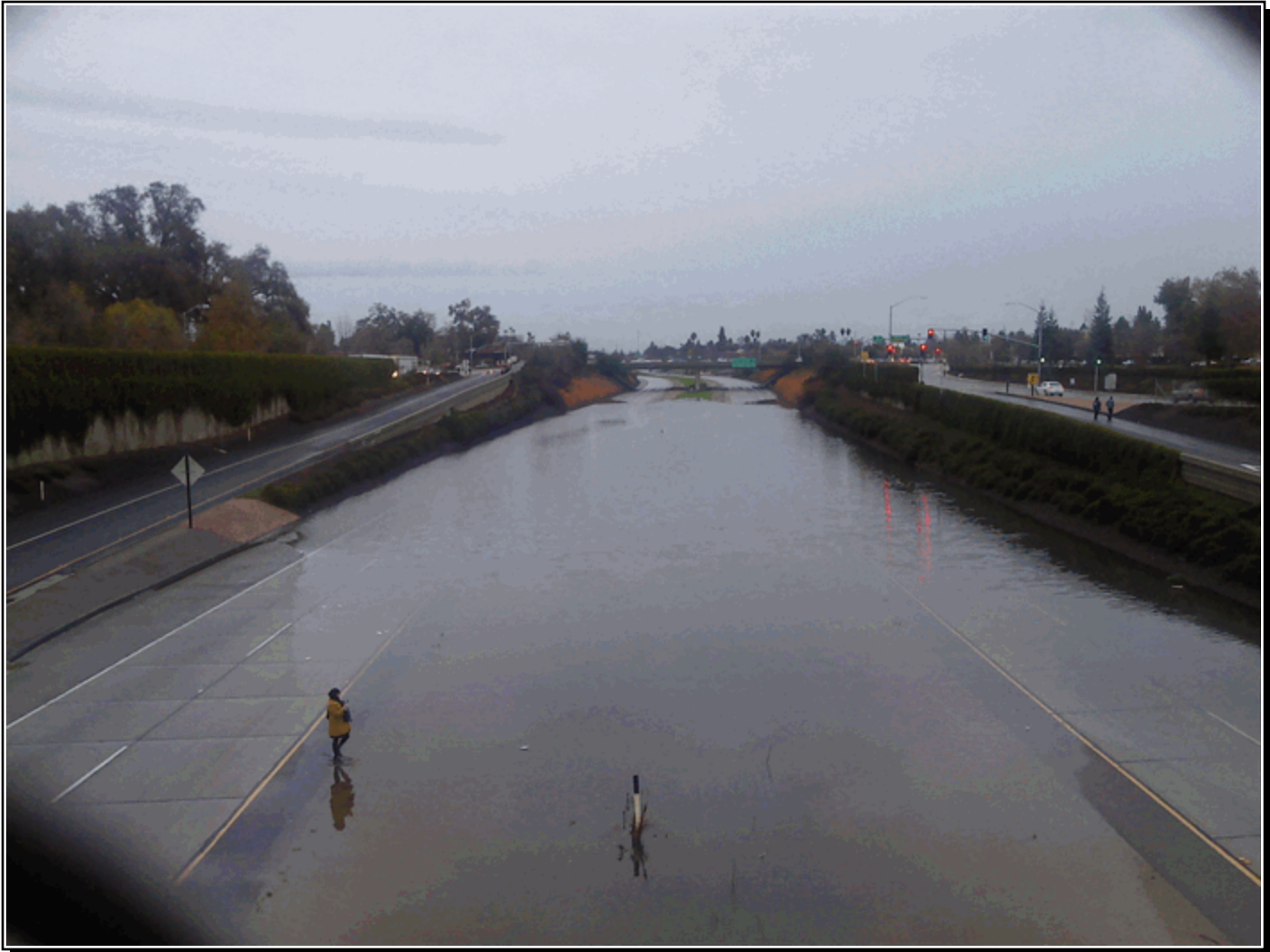
Flooding of Highway 198 through Visalia occurred on December 19th. This is the principal freeway through the city. Image courtesy NWS Hanford, CA.
