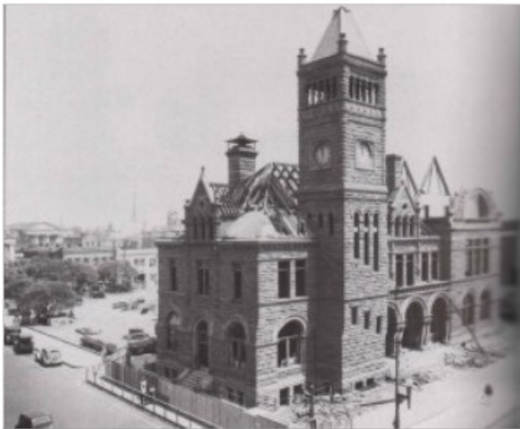
U.S. Post Office building slowly demolished beginning in 1936.
