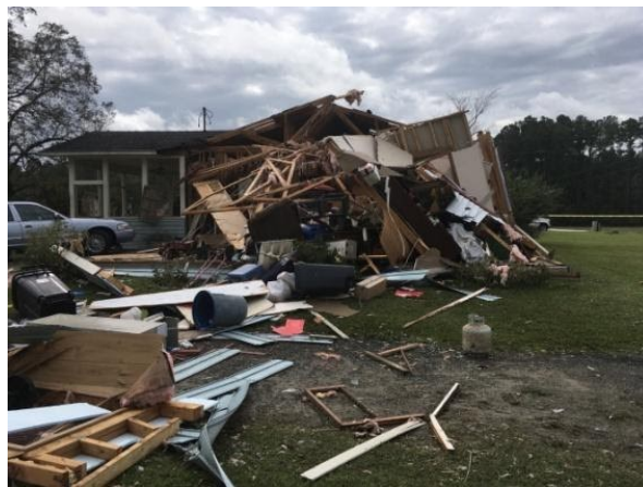
Damage in Conway, SC from a confirmed EF1 tornado on Oct. 11th, 2020.
