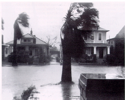
Water and High Winds Damage Galveston Texas, July 27, 1943
