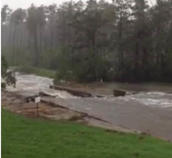
977 978 Figure 27. Spillway at Lake Hide-a-Way after heavy rainfall from Hurricane Isaac. Image is a 979 capture from video taken by Bruce Devillier. Lake elevation appears to have reached the top of 980 the concrete lining the guide channel at the time of the video. 981
