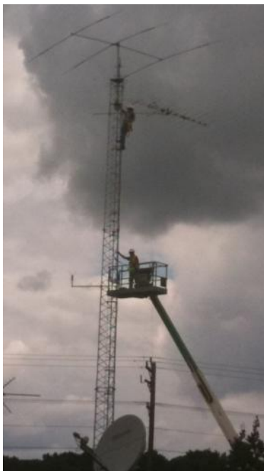
ET's Climbing the Antenna Outside the Forecast Office
