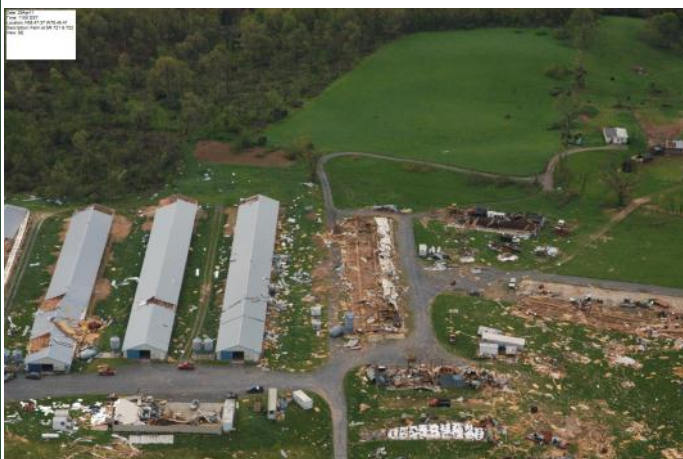
Shenandoah County Damage to a Poultry House
