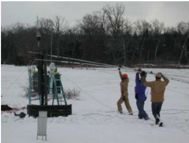
Equipment setup in the snow (photo by Leila)
