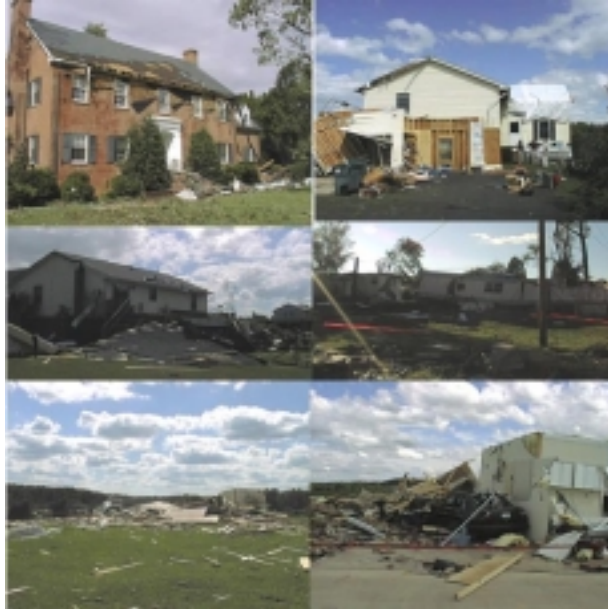
Damage from tornadoes in Culpeper and Fauquier Counties (photos by Steven Zubrick-NWS) Top row left: A two-story porch was ripped off a house 1/2 mile west of The Plains; right: An attached garage was ripped off a house in Jeffersonton; 2nd row left: Pieces of a church roof were blown a quarter mile and ended up in the front yard of the house that lost its garage; right: At Ponderosa Trailer Court in Jeffersonton, three trailers were destroyed and two people were injured by flying debris; Bottom left: A two story brick house (similar to the one pictured top left) was flattened by the tornado and debris was widespread; right: A picture of what remains of the house including a piece of the kitchen that ended up where the garage used to be.
