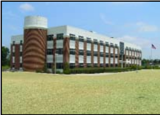
Office location of both the NWS Middle Atlantic River Forecast Center and the State College Weather Forecast Office.
