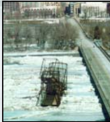
Icy floodwaters destroy the old Walnut Street Bridge in Harrisburg, PA, in January 1996.
