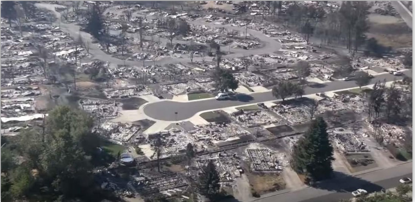
Devastation from the Almeda Drive Fire in the area of Phoenix and Talent in southern Oregon. Screenshot from video shot by Jackson County on September 8, 2020.
