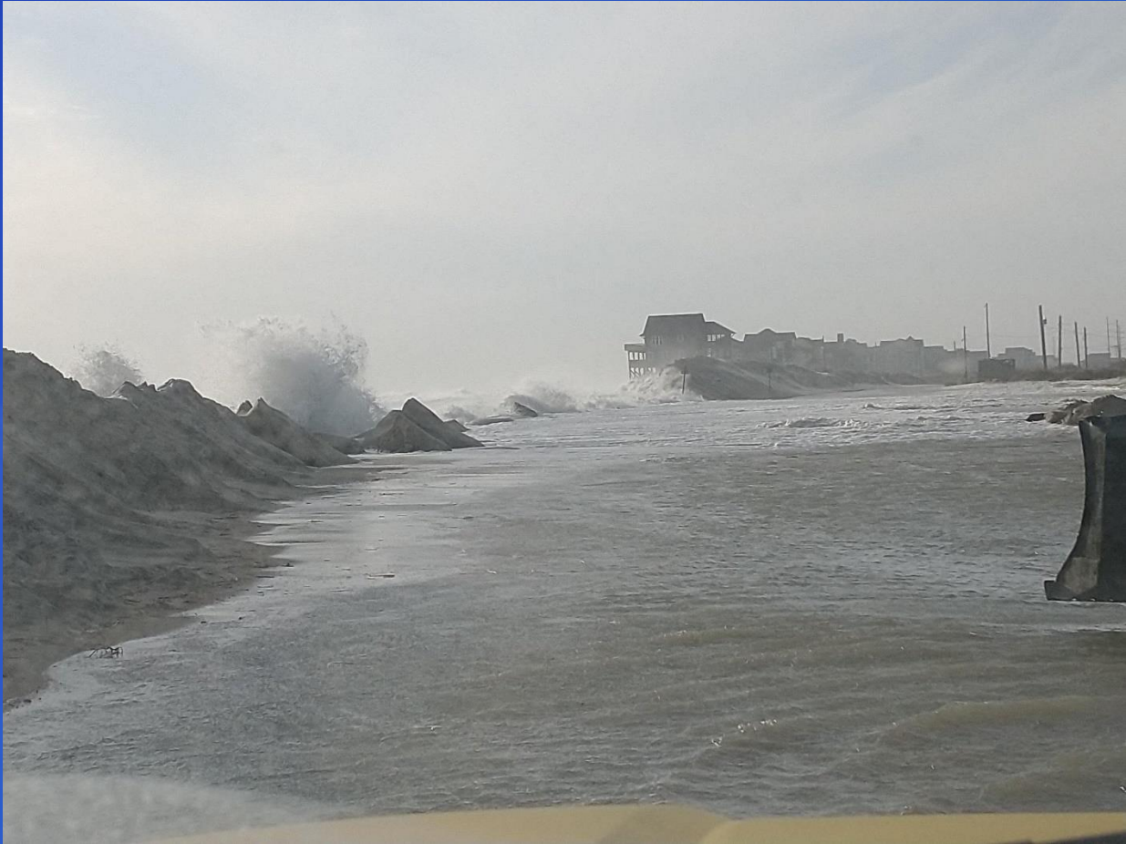
Ocean overwash north of Rodanthe on Highway 12 on November 7, 2021. Image courtesy of the NC Dept. of Transportation.
