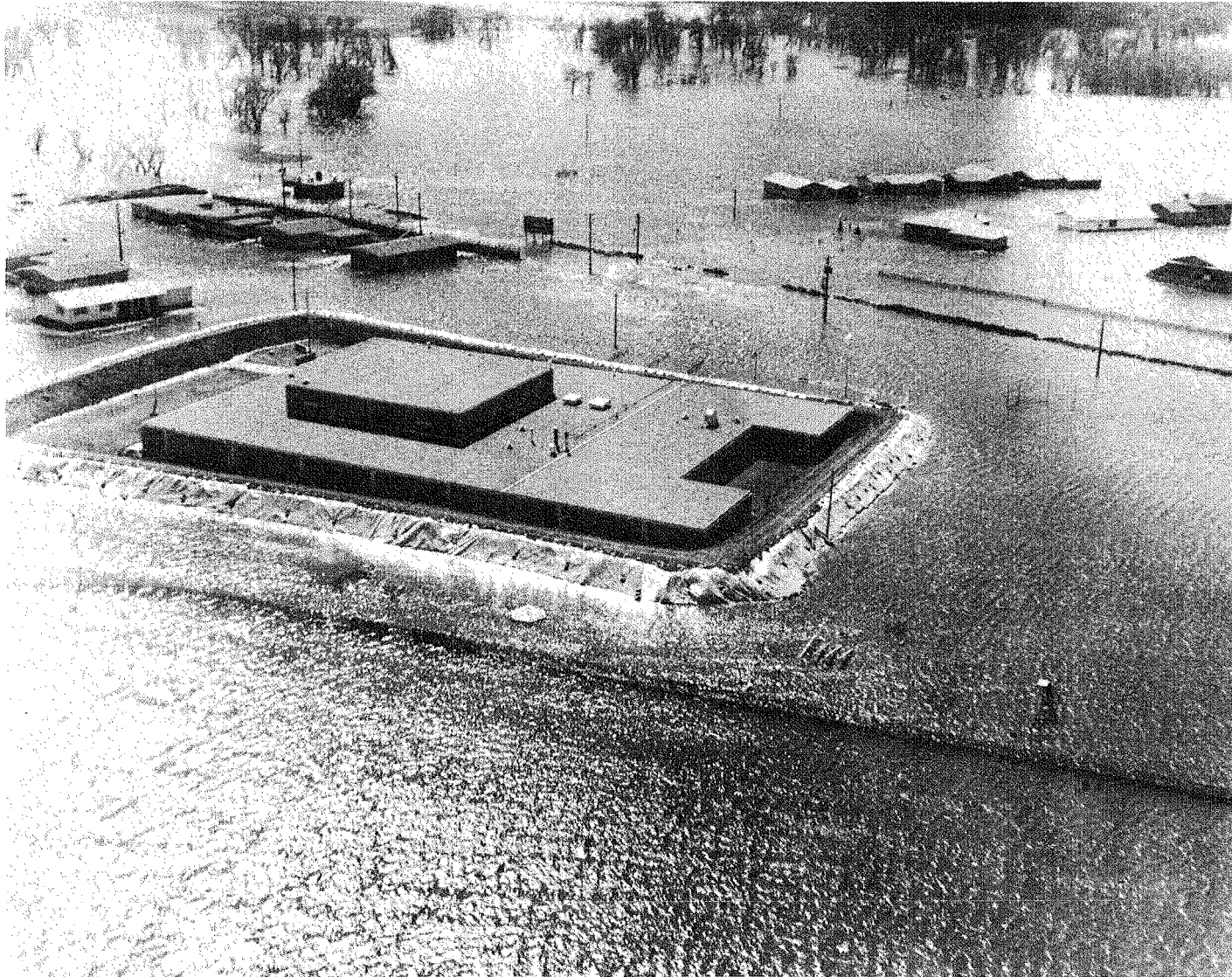
School in Minot, N. Dak., protected from flood waters by emergency dikes erected on basis of early warnings. Photographed by North Dakota National Guard on April 11, 1969, 8 days before flood crested.
