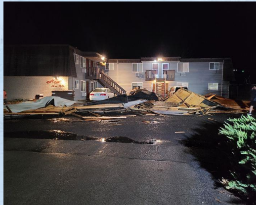
Wind damage near downtown Pendleton on January 13 th due to a strong cold front.
