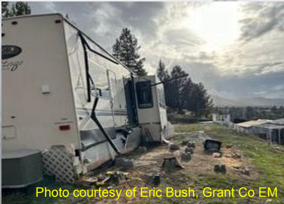
EF0 tornado damage near John Day, OR
